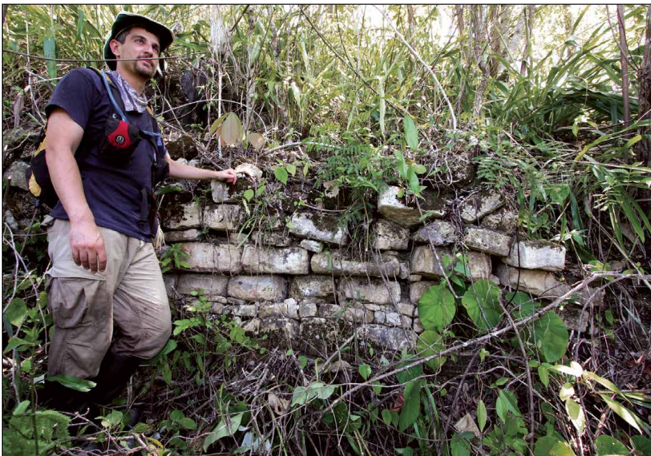
Figure 21. Close-up of intact terrace wall of Structure 1, Laguna Oscura. Photo: Andrew Scherer.
